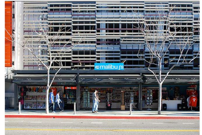
**Figure 7** This garage uses architectural elements to screen cars at the upper floors while providing retail at the ground floor. Photo Credit John Edward Linden.
